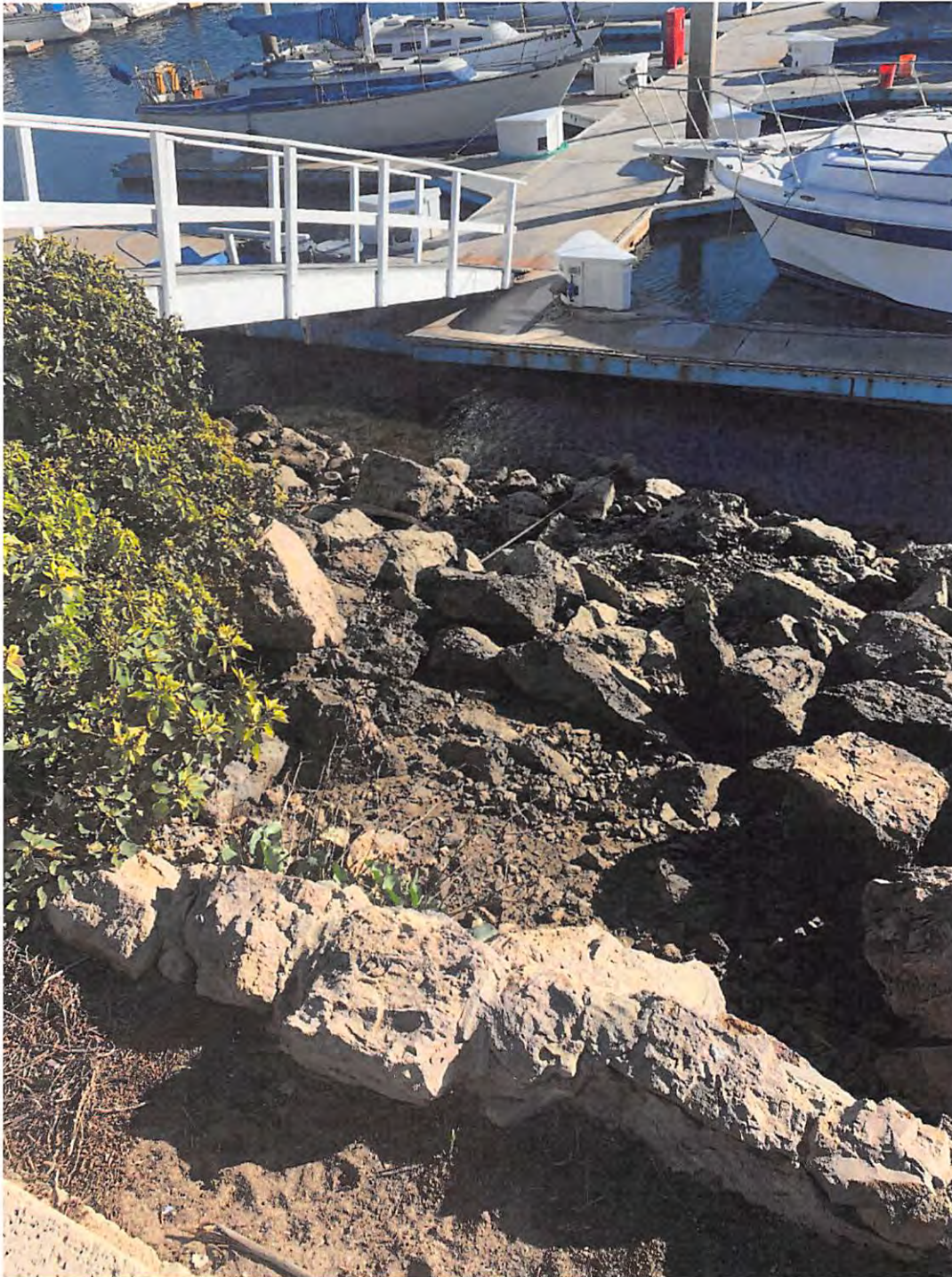
Photo showing loss of revetment stone at south end of peninsula near Peninsula Yacht Marina gangway.
