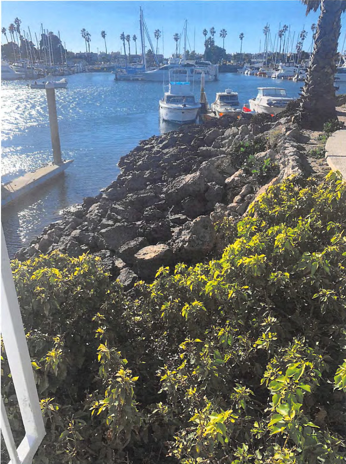
Western corner (looking west) at end of peninsula shows rock revetment sluffing from bank into the harbor.
