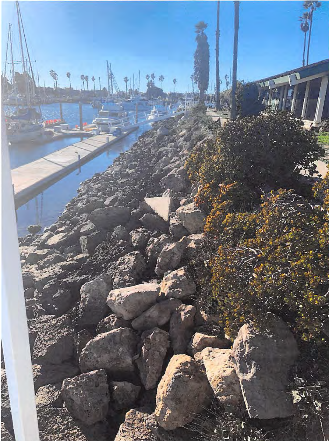
Photo taken at southeast corner of peninsula looking west at southern edge shows extent of rock revetment movement from slope into the harbor.
